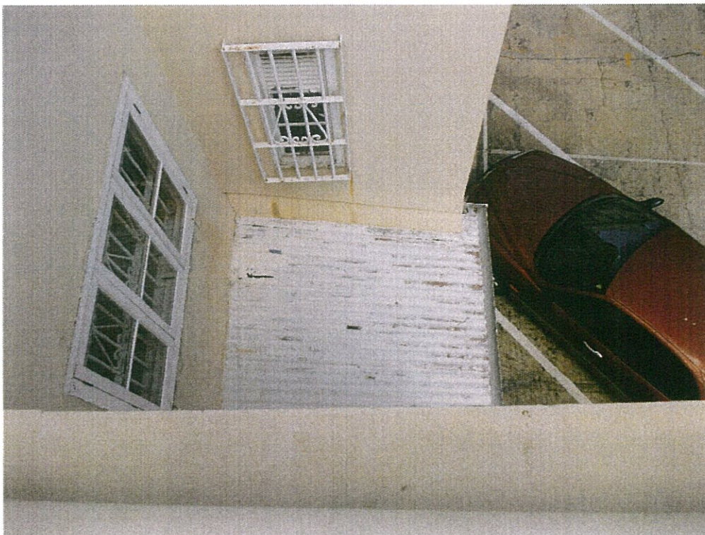
Fig 4 Looking down onto asbestos cement roof sheets
