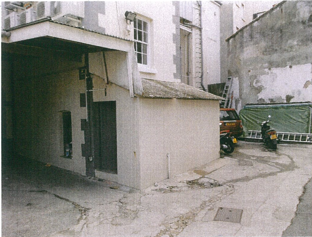
Fig 5 Single storey lean too with asbestos cement roofing sheets
