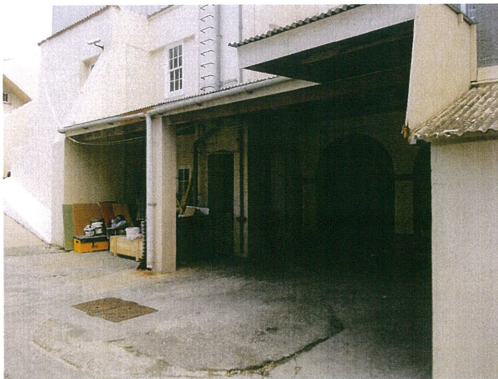
Fig 6 Timber framed canopy to be removed
