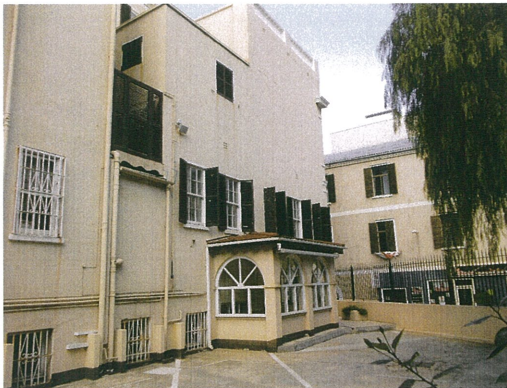
Fig 1 Part view of eastern elevation to be demolished
