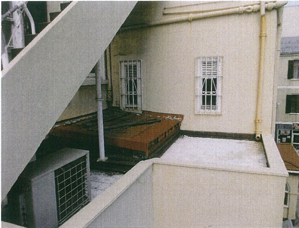
Fig 3 Looking North at extension to be demolished
